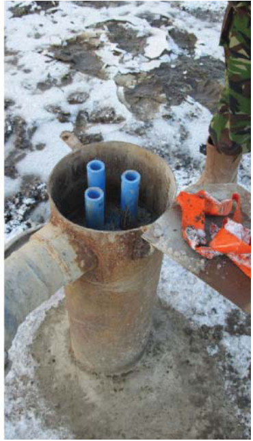
Figure 4.13 This borehole was drilled to a depth of 75 m near Morpeth in Northumberland in the Stainmore Formation at the top of the Namurian Group. Three piezometer pipes were added with response zones at 75–54 m, 38–29 m and 20–11 m. Each piezometer was surrounded by gravel and the rest of the borehole was filled with a sand/bentonite mixture. The left-hand drawing shows the relationship between the piezometer and geology, with different water levels in each piezometer. The water level in the highest piezometer is above that in the next one down; confusingly, that in the deepest one is above that in the highest one. The right-hand photograph shows the surface arrangement.
